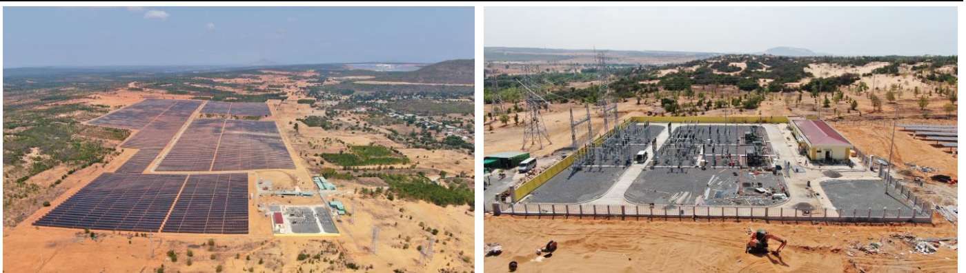
Figure 32: Construction progress at Hong Phong 4 as of early May, 2019
